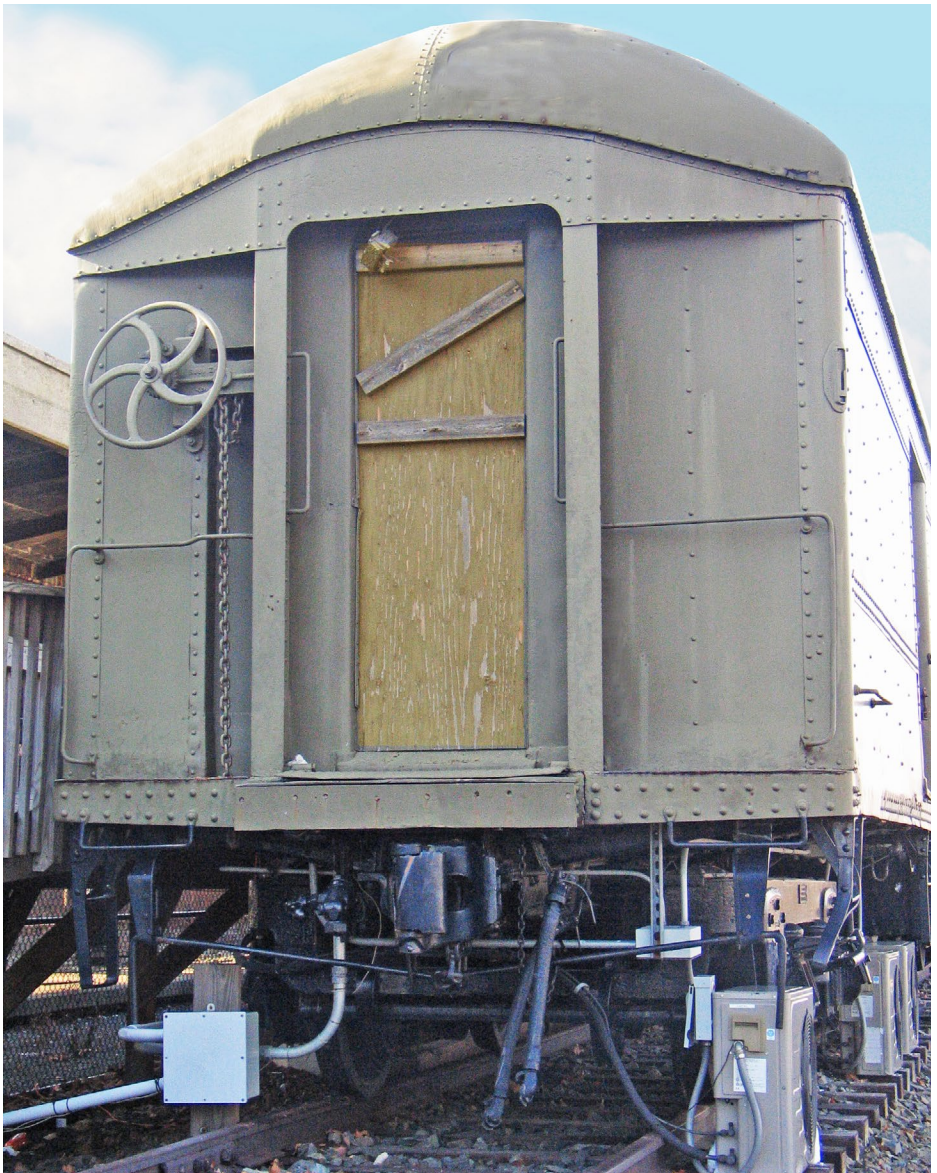
8. Blind end of Lackawanna baggage car, a typical arrangement similar to SP 80-BH-1 cars. The end sheets of the car are flat and are mounted to the inside of the collision posts framing the door.
