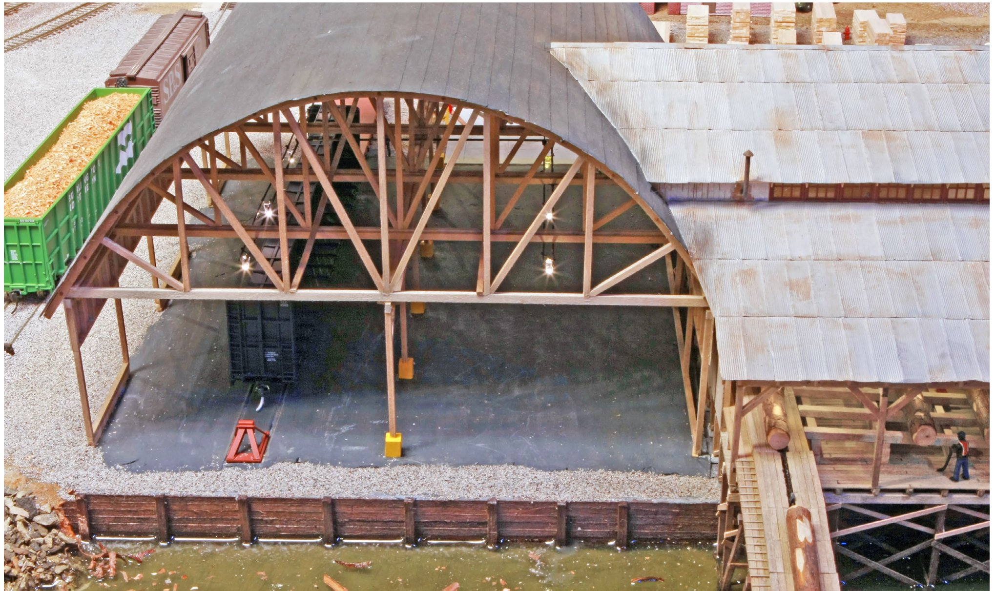
11. Next, is this close-up of the lumber mill's curved-roof loading area. This curved truss roof construction was quite common for lumber mills located in the Pacific Northwest.
