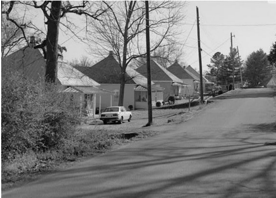
1. Five of the square-top company houses are still in use today. They have been modernized with changes in the porches and siding. HABS/HAER photo John Stewart collection
