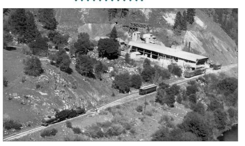
13. The locomotive on the front of a mixed train is backing into the double-ended siding at National Lead to pick up box cars loaded with either bagged or bulk barite lead. Note the combine for passengers left on the mainline and the empty tank car picked up from the facing point switch on the right/east end of the plant. Jim Boynton photo
