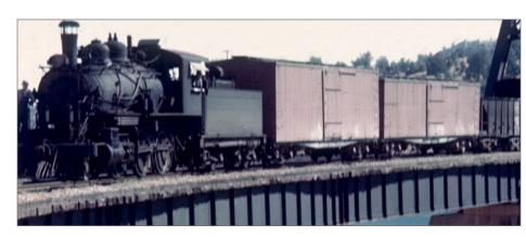
12. A close-up of a color photo of the 1945 fan trip train shows two YV Harriman box cars behind the locomotive. The first car is the taller 613 (a B-50-5 rather than one of the B-50-1/2/4 cars) while the car behind it is the 612 based on the length of the corner braces. Al Rose photo
