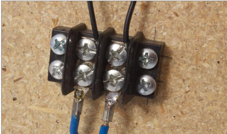
14. Large gauge (16 AWG) stranded bus connected through a barrier terminal strip to a smaller gauge (20 AWG) solid wire.
