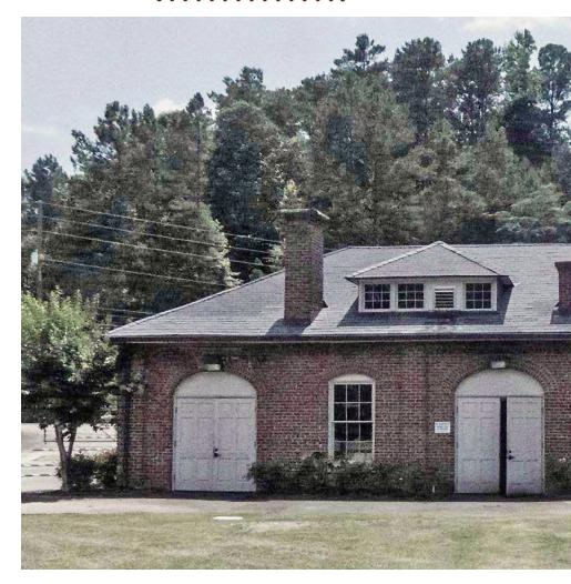
12. The locomotive, blacksmith and machine shop as it exists today. The building is 30 x 70 feet, with 20-foot walls at the eaves. The locomotive shed was in the left bay with the double doors, and the blacksmith shop was in the next bay with the double doors. To accurately model the build-ing as it was when the railroad was operating, the far right window needs to be replaced with a double door which had a square header.
