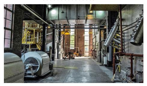
2. Inside the boiler house today. Boilers 16 & 17 are on the left, and Boiler 18 on right. The tube in front of No. 18 delivered coal to a crusher which fed fuel into the boiler's firebox. The building is a lot cleaner than when it was in operation with the coal-fired boilers. Philip Griffith photo
