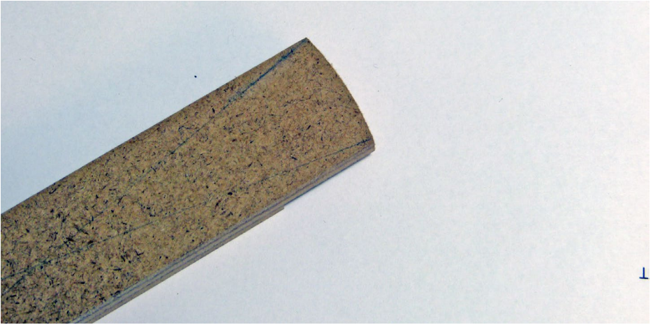
3. A close up shot of the rounded bridge edge.
