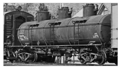
4. The Standard Tank Car Co. built this three-compartment car for the Sinclair Refining Co. in the early 1920s. Small diameter domes with elbow-mounted safety valves were common practice at that time. Note the STC underframe's distinctive bolsters. Most Sinclair cars had billboard "SINCLAIR" stenciling on their tanks, but maneuvering that large a stencil behind all the ladders on this car would have been a serious challenge.
