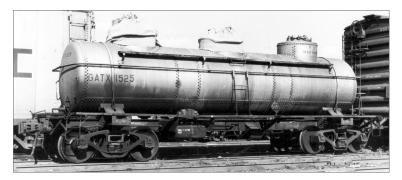
16. The tank was painted aluminum on GATX 1525 when photographed at Schiller Park IL in May 1968, so weathering is even more visible than on black cars. Note the mismatched trucks. Canvas covers over the domes, or safety valves, were often used when the tanks were empty to prevent the safety valves and manway covers from being contaminated. Bill Raia collection
