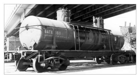
10. Built by General American in January 1926, GATX 1611 was a 6,000 gallon two- compartment car. Again, note the small diameter domes with safety valves on elbows. Oil spills like those shown here were common when cars were being loaded. This car was still in revenue service in the early 1970s when photographed at Bakersfield, CA.
