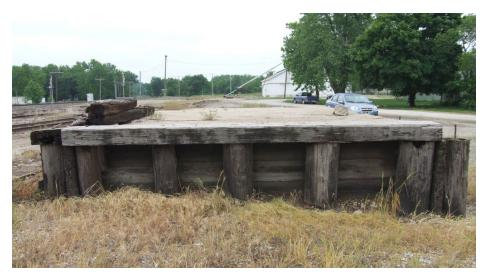
5. The platform end of the dock, looking south. Note the heavy timbers used as a top chord, and also where they are missing on the dock's sides. Also notice the heavy round poles used to support the structure. May, 2008. Photo by Jared Harper
