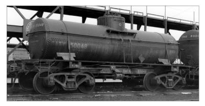
2. 4,000 gallon tank cars were more common. This one, built by General American in January 1928, was still in revenue service when photographed at Los Angeles in the early 1970s. Note the two-horizontal-section tank, the substantial wood blocks between the bolsters and small diameter tank, and the underframe design which, with minor revisions, was later designated by GATC as the Type 30.
