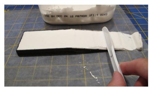
15. Once the frame was filled I used a plastic knife to gently level the Hydrocal on top of the ramp.
