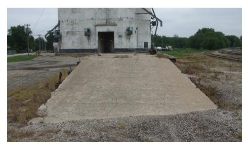
4. The ramp end of the loading dock, looking north. The interior of the entire structure was filled with sand and a concrete liner applied on top of the sand. May, 2008. Photo by Jared Harper
