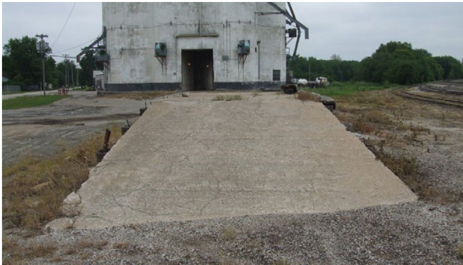
4. The ramp end of the loading dock, looking north. The interior of the entire structure was filled with sand and a concrete liner applied on top of the sand. May, 2008. Photo by Jared Harper
