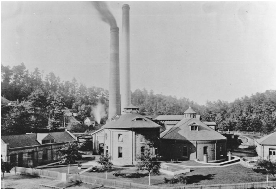
2. The Cahaba River Pumping Station of the Birmingham Water Works. Larry Smith Collection
