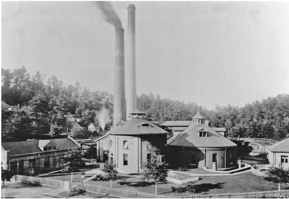
2. The Cahaba River Pumping Station of the Birmingham Water Works. Larry Smith Collection
