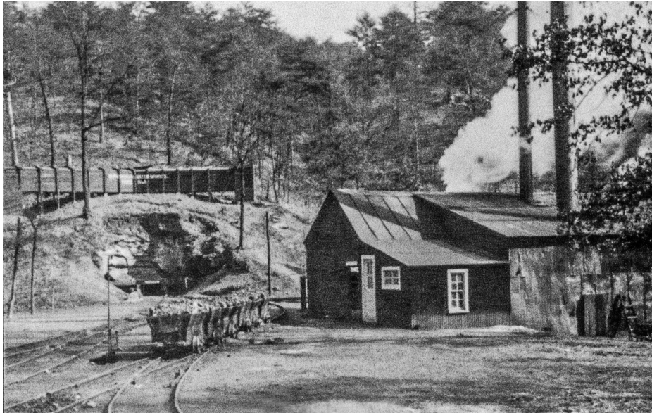
4. The Merkle Mine showing the trackage and the hoist house. The entrance can be seen to the left of the tiny mine cars. Phillip Griffith Collection
