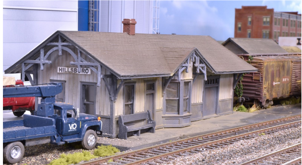
20. Another view of the old V&O station at Hillsboro, now being used by the maintenance of way department.
