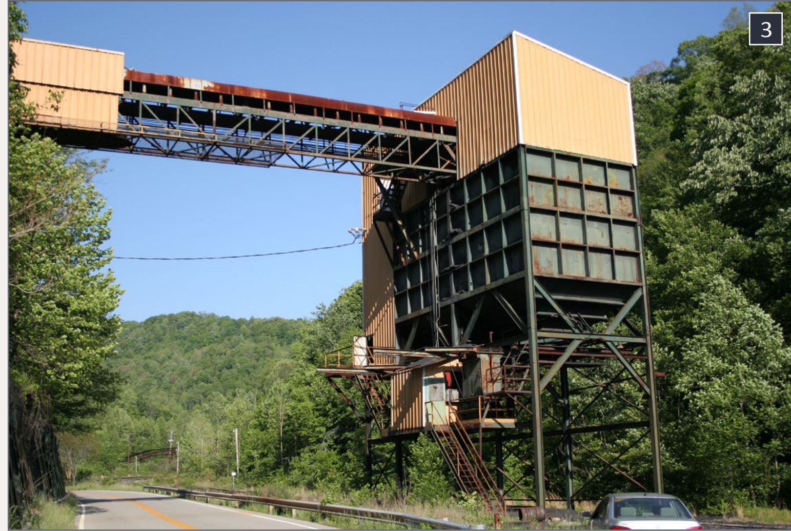
3. A fast loader that resembles the Walthers Flood Loader kit. This facility is Alamo-Harber Coal at Alamo, KY.
