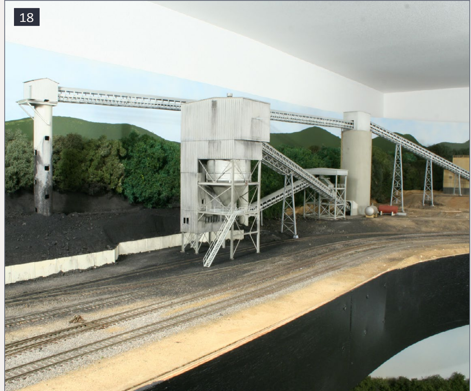
18. Coal stacker, fast loader, transfer building, concrete storage silo, conveyors, and main preparation building.
