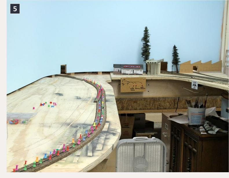
5. With the sub-roadbed in place, I started to glue down cork roadbed. This area of Browning is on a 1% grade, descending toward the backdrop.
