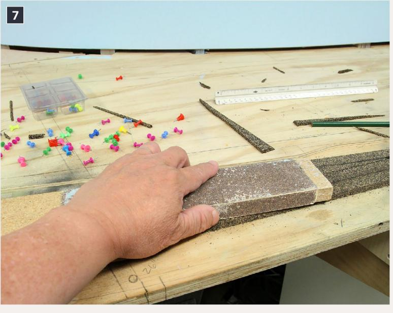
7. Sanding gets rid of high spots and rough edges. Sanding with a long sanding block reduces side-to-side and up-and-down dipsy-doodles in the cork roadbed.
