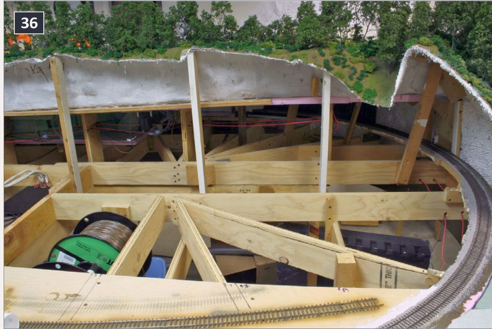
36. The joist marks were extended onto the plywood sub-roadbed so that I could still know where the joists were when the green foam was installed.
