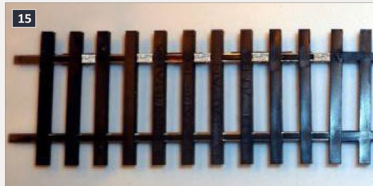
15. Cutting away the section between the ties.
