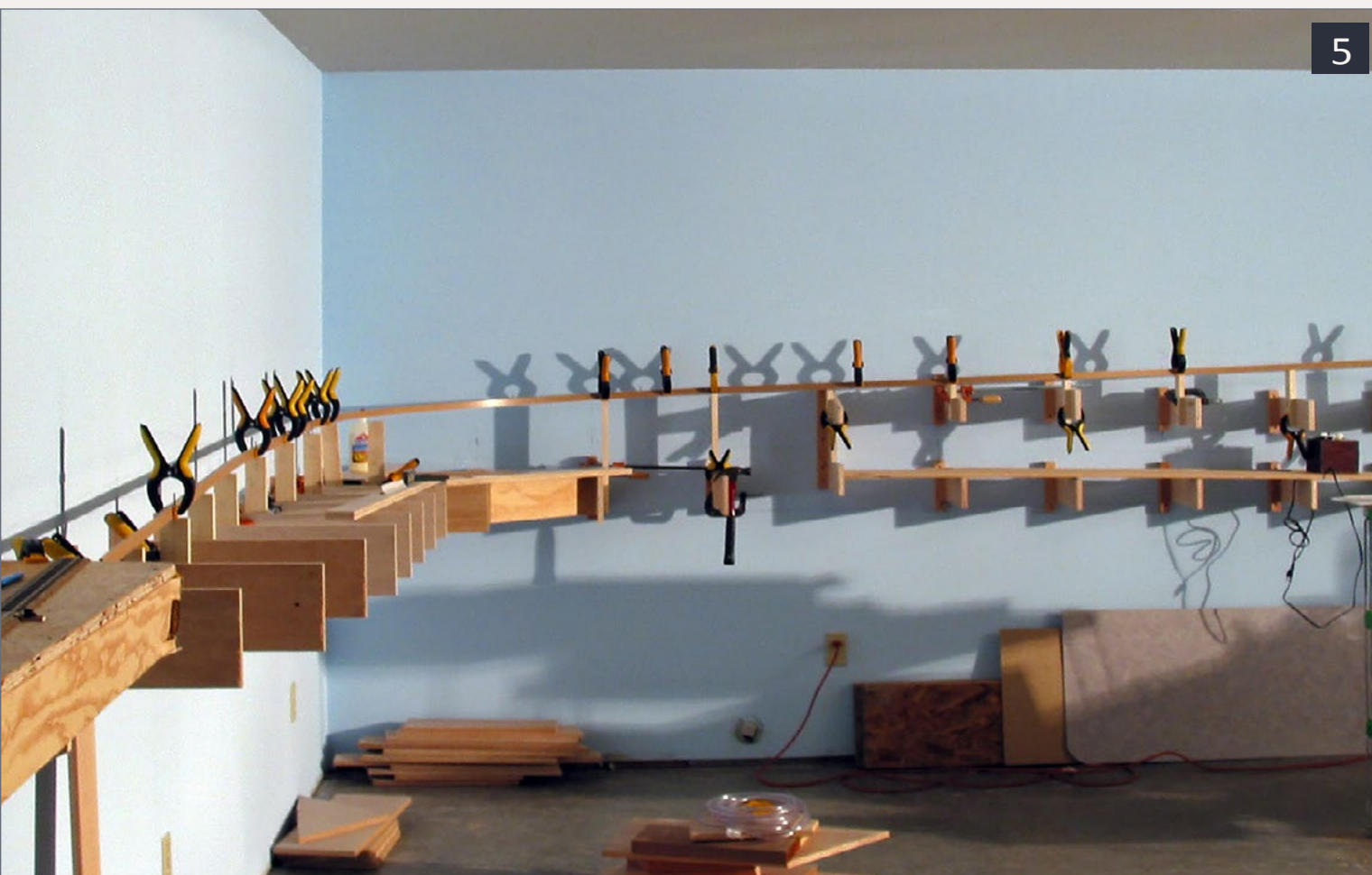
5: In the beginning was Mill Bend (the recycled Mill City from the previous layout), nearest on the extreme left. In mid-January 2004, Masonite spline roadbed installation was going gangbusters heading for Oakhill (top) and Redland (bottom). Clamping all those splines needs strong wrists!
