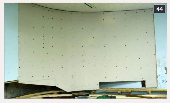
44: I smartened-up for the drywall portion and waited until Train Night when my friend Dave Santos could come over and help me hang this piece of "flexible" drywall. It's in quotations because it's not nearly as flexible as I thought it would be, and it actually snapped in a couple of places. I should have soaked it more thoroughly, but I was in a hurry.
