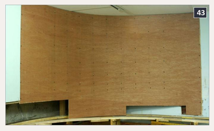
43: Here the lauan <sup>1</sup>/<sub>4</sub>" plywood is screwed in place. It's a two-man job, but I did it myself! The many screws ensure against pull-out, as the panel is under a fair amount of stress.
