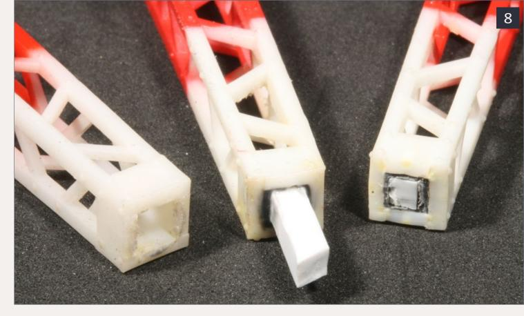
8: A short length of Evergreen #105, .100 x .100" styrene strip into the top of the tower and cut it flush. This will fill the large hole.
