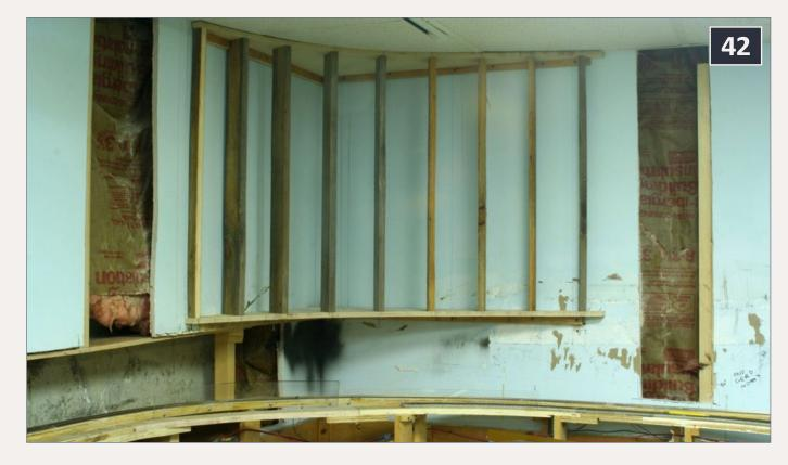
42: Here's the assembled curve corner stud assembly in place. Note that it fits up flush to the ceiling but does not attach to it in any way, in case I needed access to any-thing above the tiles.
