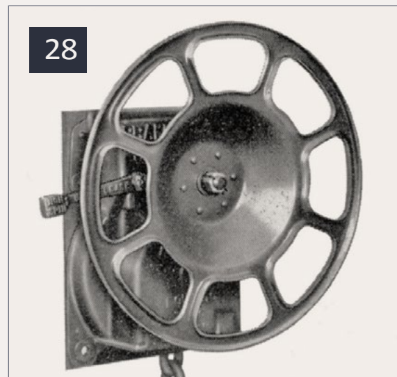
27. Ajax model IP80 with release lever at the lower left.
