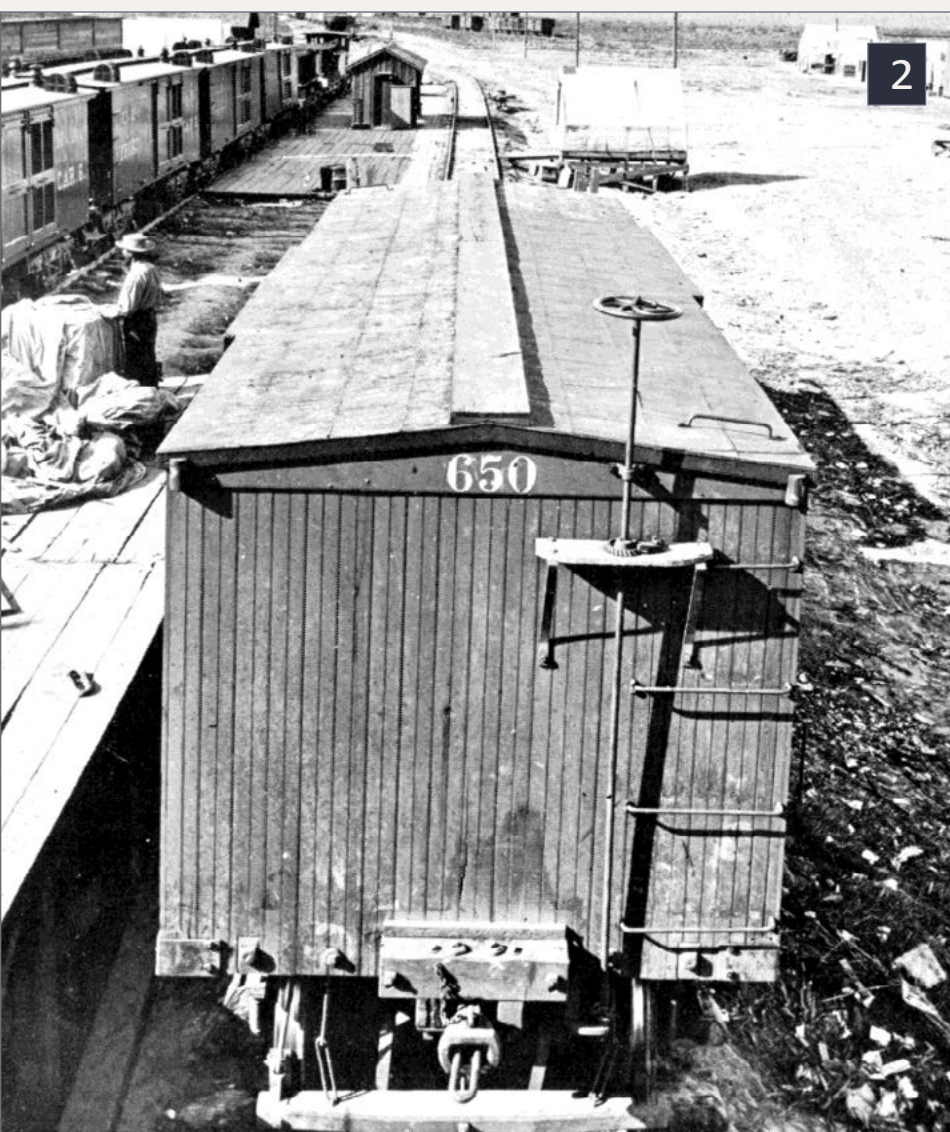
2. Vertical "stem-winder" hand brake from 1869.
