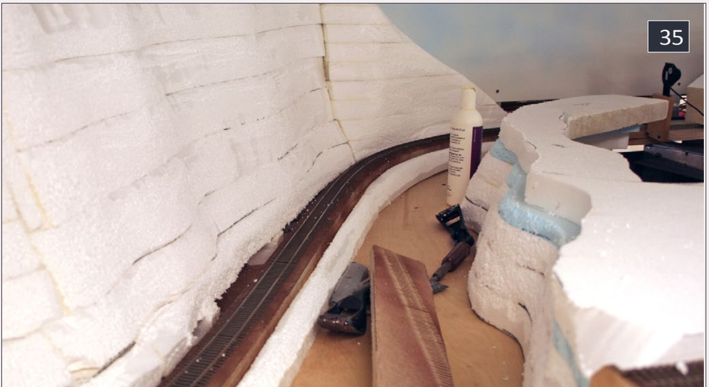
35: Foam-board construction at Guest River. Rough shaping and clean up is completed. The L&N mainline follows the river through here.
