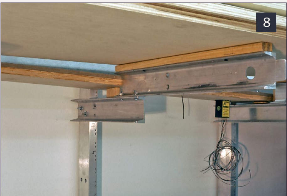
8: This photo shows the framework modification allowing for different track levels. This type of construction is not possible with wood framing, but with the metal members it is no problem. I used ¼" x 1" long bolts, nuts, and washers for my standard.
