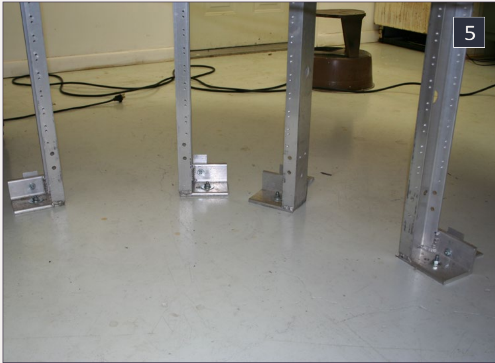
5: View of the inside curved section of vertical aluminum posts' floor mounting. Every leg is anchored to the floor providing a very sturdy layout base.
