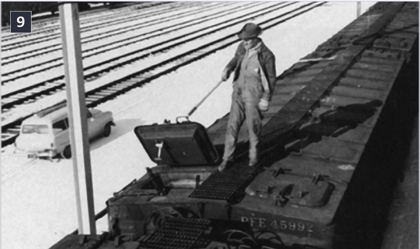
9-10: These two photos at Ogden in 1962 illustrate part of the icing process. At left, a workman is opening ice hatches, and at right the estimator chawks an amount of ice needed to top off the bunker (in hundredweights) on the hatch plug. The same amount would be noted on the clipboard in his left hand for that car number. This chalking operation is for the operator of the icing machine moving along the deck. Chalking was not needed in the days of icing with hand tools. –both photos, PFE, courtesy CSRM.
