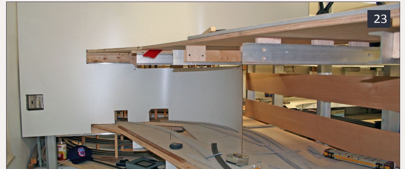
23: The finished side of the hardboard backdrop as it is being placed on the mid and upper level. By staggering the joints between the plywood strips and the backdrop, I don't have to worry about any unsupported joints moving at some point in the future.
