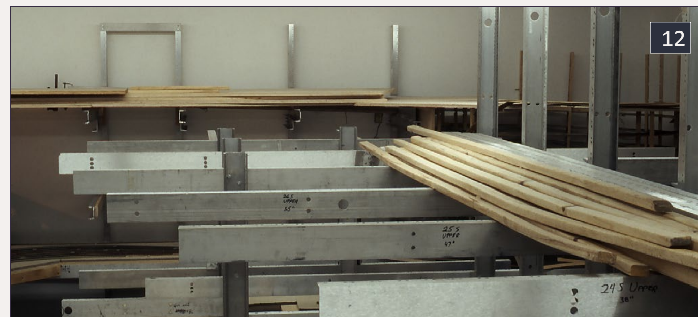
12: The end of the peninsula from the upper level. Note the good 1x2 lumber! One of the major advantages of the metal framing is I don't have to worry about warped lumber.
