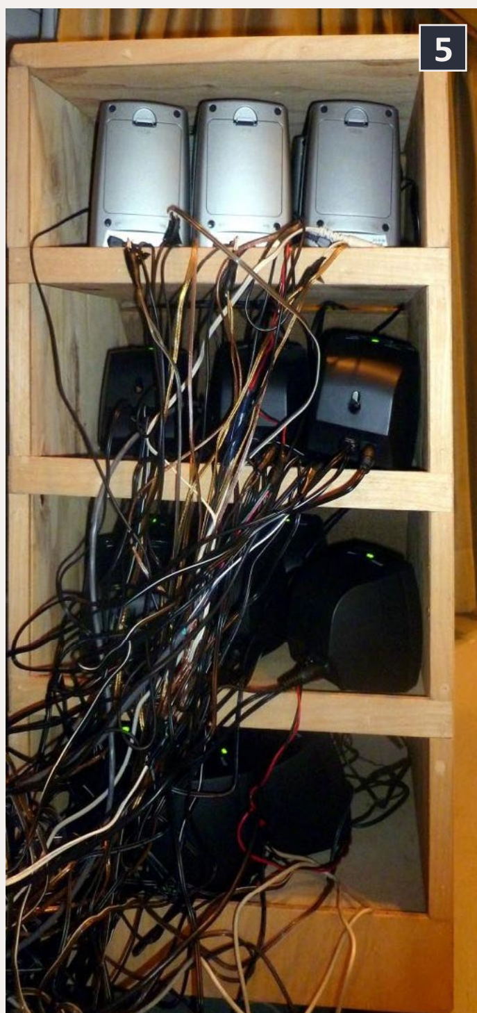
5: Here is the back side of the cabinet that holds the speakers with amplifiers and controls.
