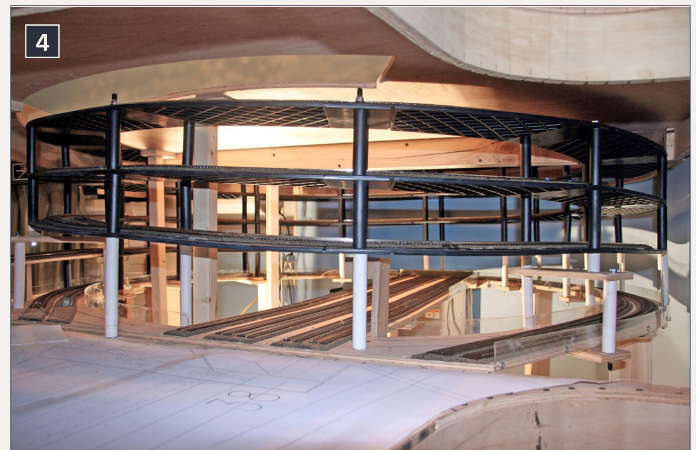
4: The helix at Shreveport Union Station.
