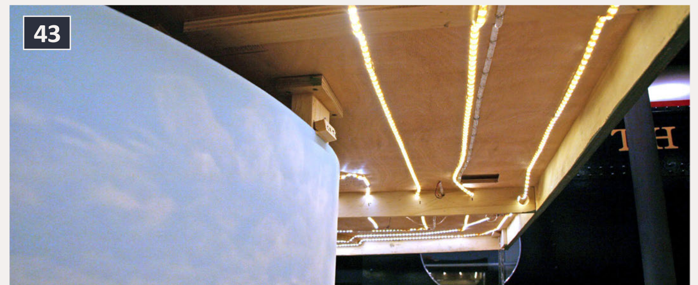
43: Warm white LED strips 6" apart to light the lower deck.
