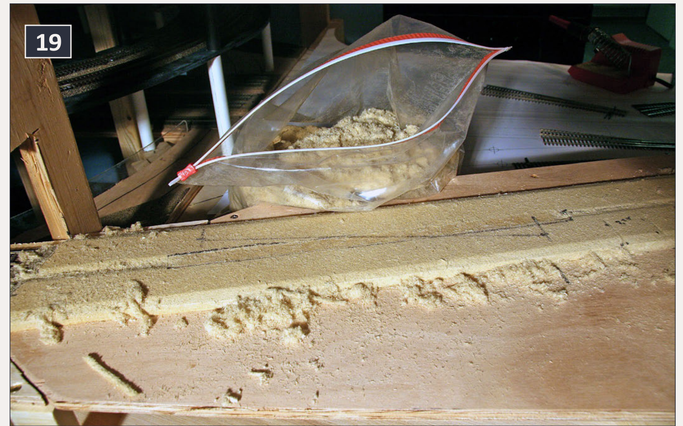
19: Fill the gaps with Celotex sawdust.
