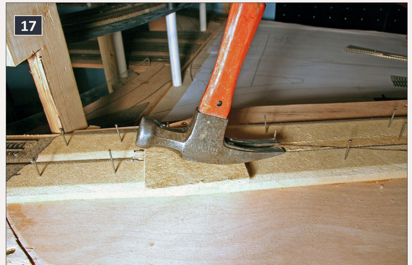
17: Removing the nails.
